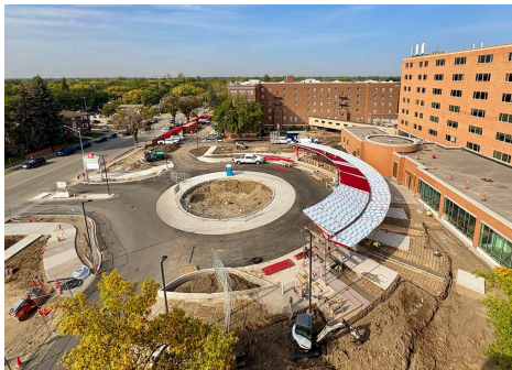
Exterior landscape work in progress
